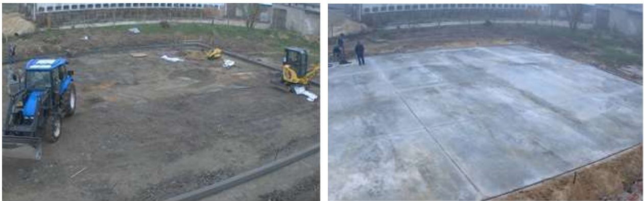
Figure 2: Construction of infrastructure; container & manipulation surface
